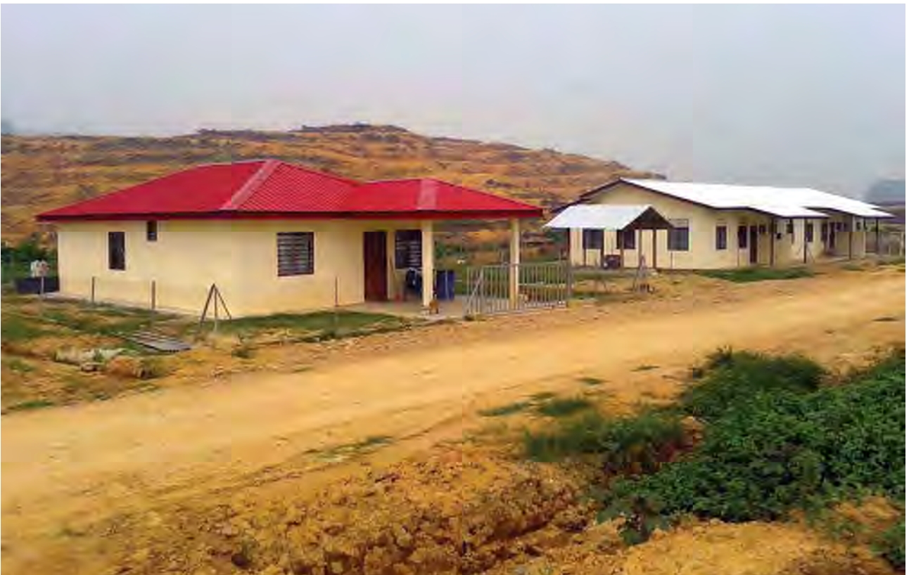
Kuala Pergau Estate Workers Quarter and Staff Bungalow.
