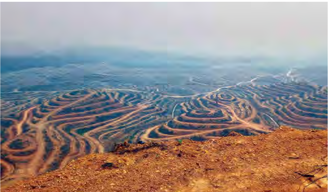
Kuala Pergau Estate - Terracing of Slopes.
