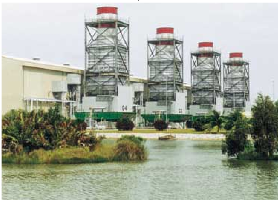
Port Dickson Power's 440MW peaking plant power station at Tanjung Gemuk, Negeri Sembilan Sesen janakuasa loji puncak 440MW milik Port Dickson Power di Tanjung Gemuk, Negeri Sembilan
